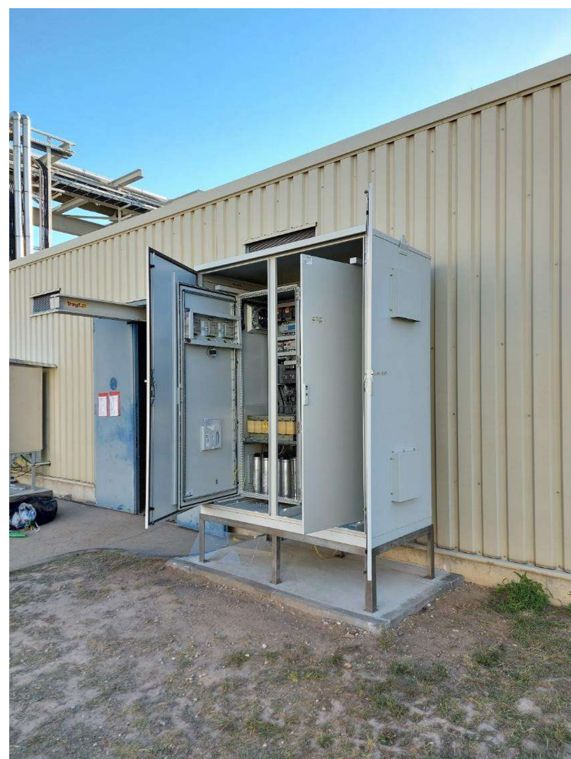
Customised interventions banks and reactors designed for groups of smaller electric loads Dynamic filter behaviour based on operating conditions (i.e. combinations of loads)
