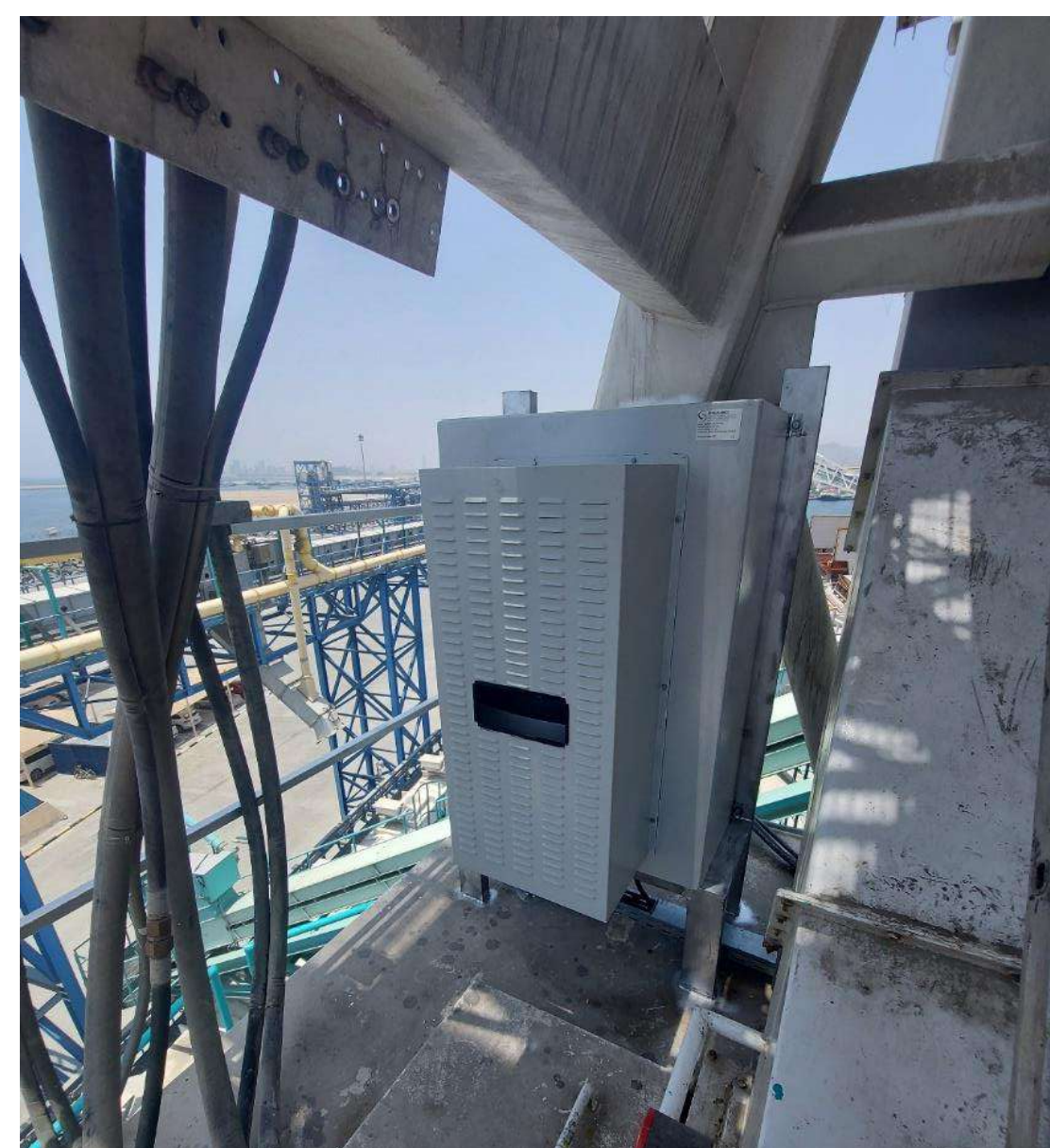
Passive Harmonic Filter , mitigates reactive power and current harmonics (lower levels of harmonics)
