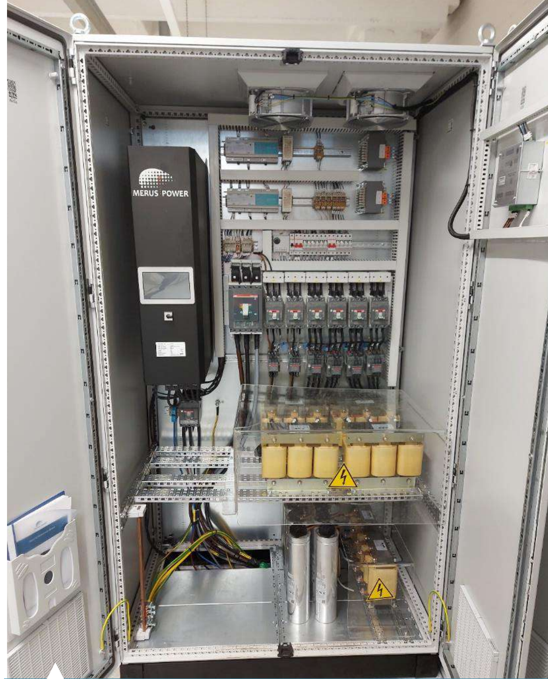
Hybrid System , Active and Passive Harmonic filters built in the same enclosures
