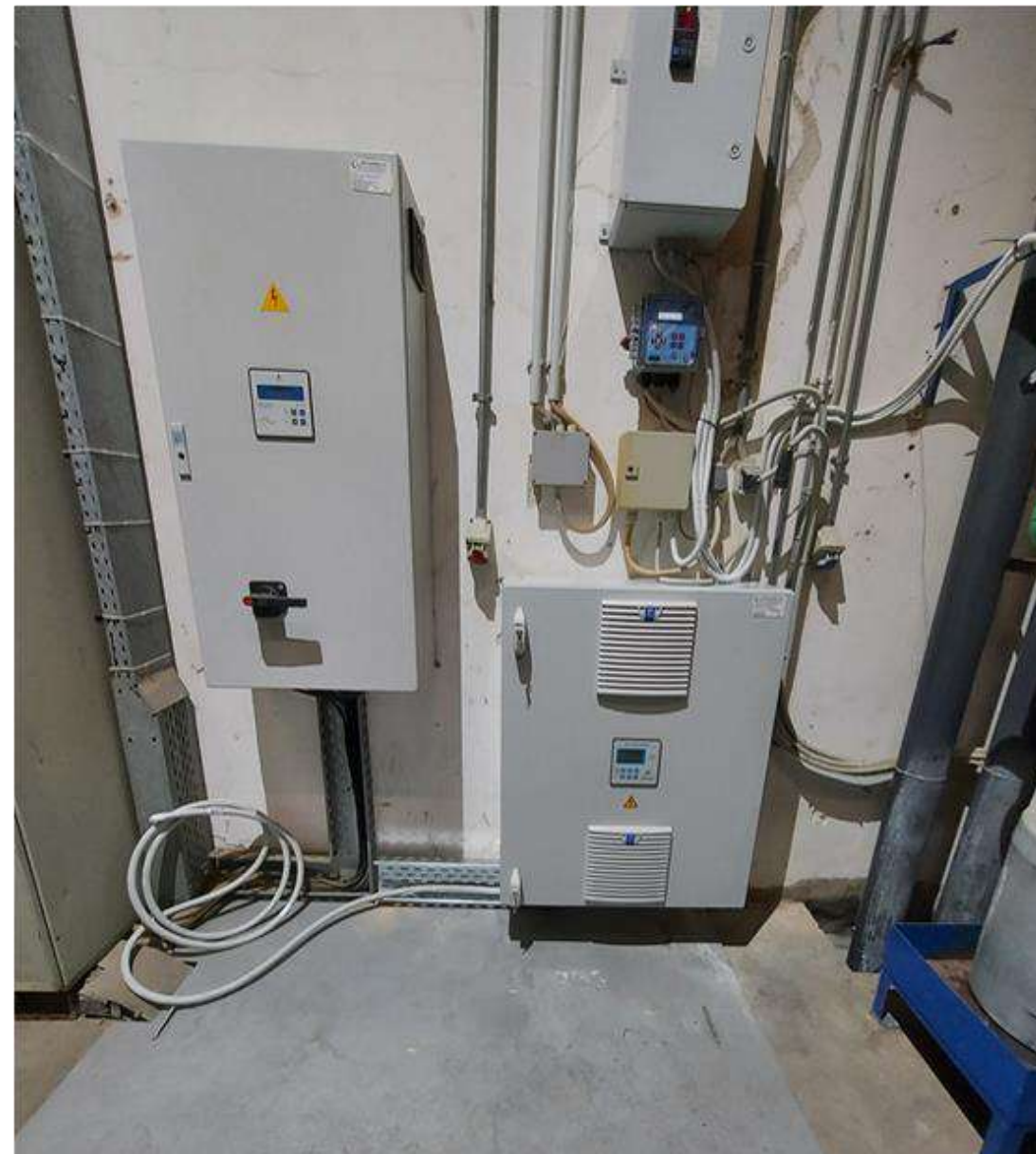
Hybrid System , Active and Passive Harmonic filters built in the same enclosures
