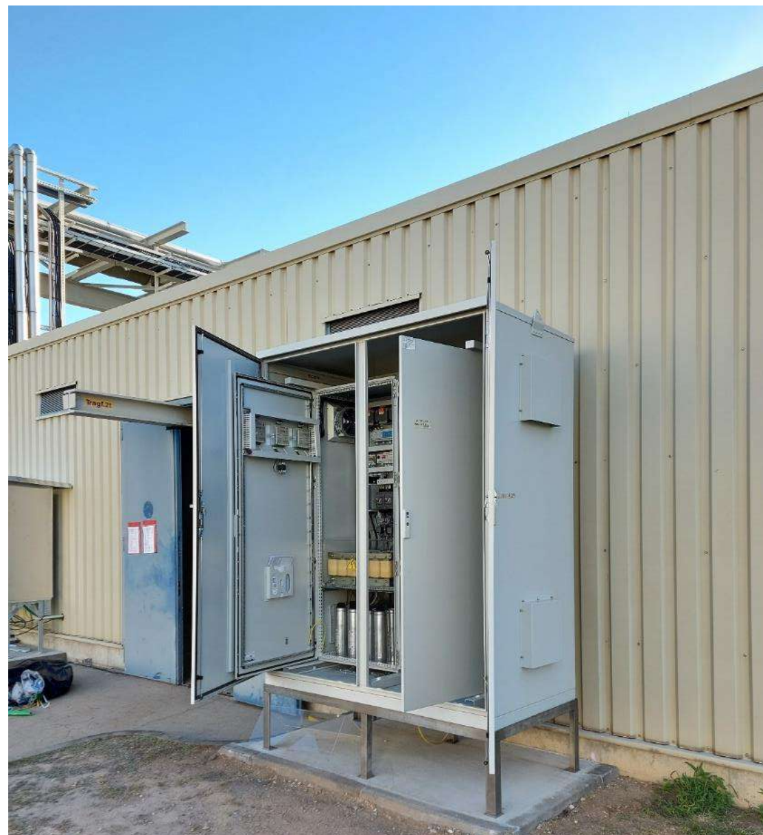
Active Harmonic Filter , mitigates current and voltage harmonics
