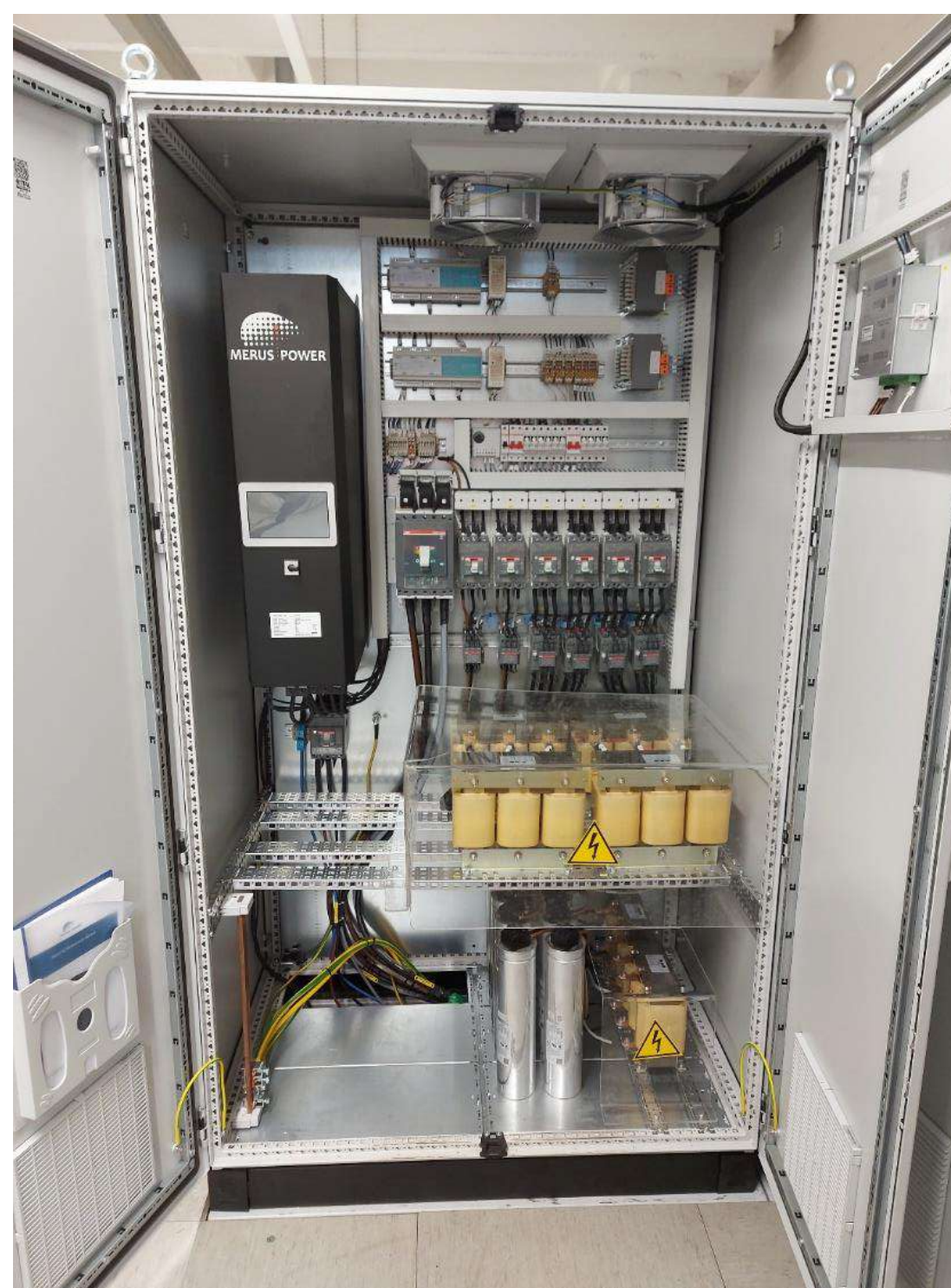
Customised interventions banks and reactors designed for groups of smaller electric loads Dynamic filter behaviour based on operating conditions (i.e. combinations of loads)
